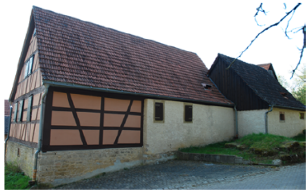
Figure 1: Image of a timber-framed building, where the detection of the vertical direction in image space will probably fail.
