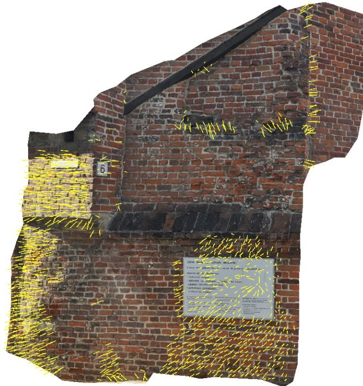
Figure 5.28: Positions and directions of 1117 unknowns in the mesh marked in yellow at pyramid level 0.
