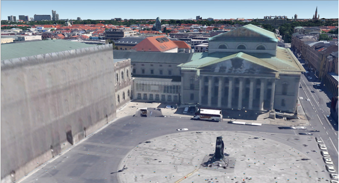
Figure 1.4.: Screenshot of a view in Google Earth from the opera in Munich. The simple model of the building comprises a small set of planes. The simplicity affords fast rendering of large scenes but discards complex geometries. Details such as the pillars are mapped onto a plane. © 2014 Google, © 2014 DigitalGlobe
