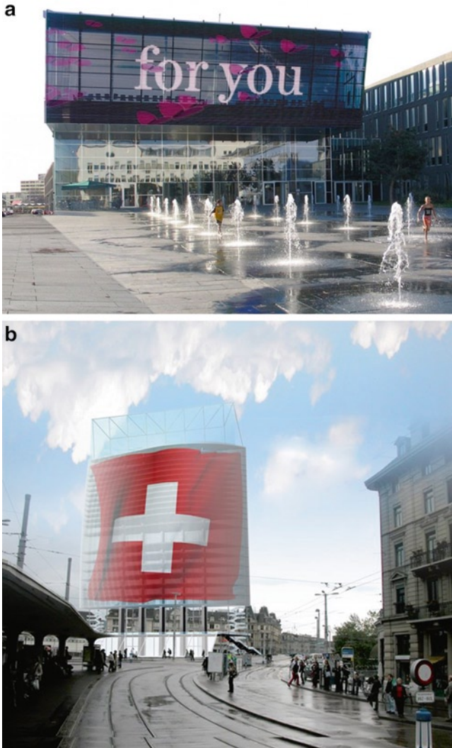
Fig. 2.8 Media facades – light and media technology embedded in architectural facades – create an interface between the architectural and urban space on one side, the digital and narrative space on the other side (a) T-Mobile Headquarters, Bonn, the first permanent media facades worldwide; (b) Transparent panel structure with LEDs for Helmut Jahn’s concept of a new convention center in Zurich (Photo & rendering: © ag4 mediatecture company, Köln)
