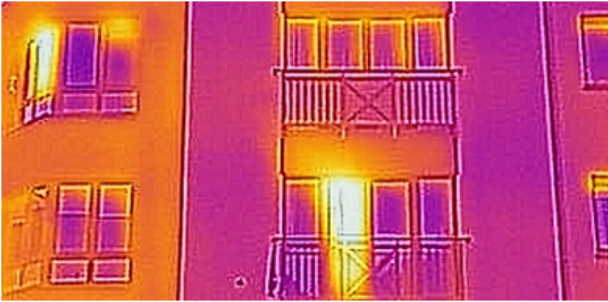
Figure 3.9: House from outside to identify opened windows or doors.
